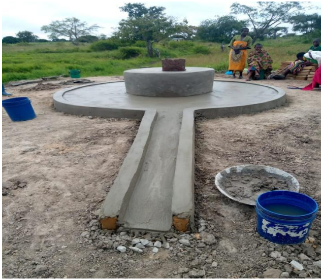
Photo 2: From Left Side Shows the construction of a Shallow well at Nambubi Village Next Shows a charcoal Dam implemented at Isenengeja Village both are at the finishing level at Mbogwe DC
